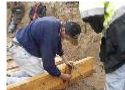
Andrew Burgess secures the plank with the chain binding them all together.
